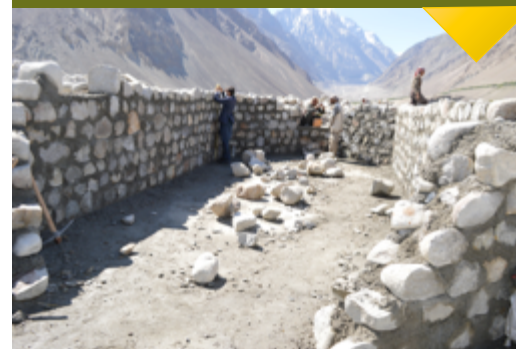
A sedimentation flushing house constructed at Qala-e Panja village Wakhan
